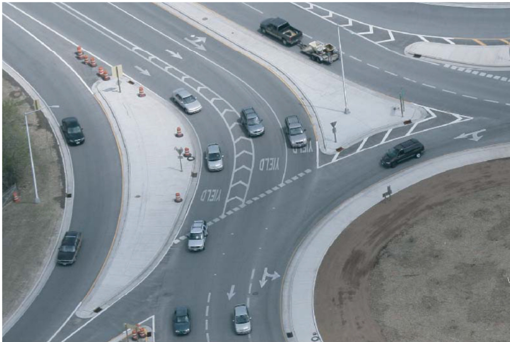
Figure 7: Pavement Markings on Roundabout Approach
