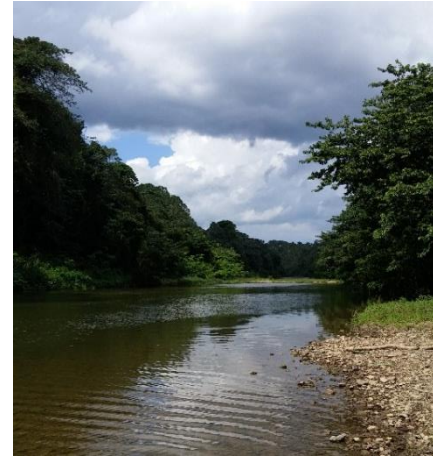
Figure 18: Photo of the dam site.
