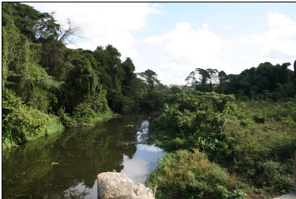
Figure 3. Photo of the proposed dam site.
