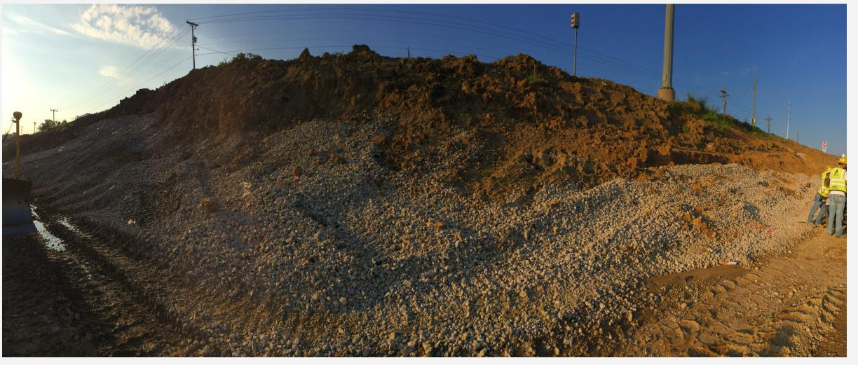
The analysis of the slope indicated that the slope A Texas Cone Penetrometer test was completed and failure was located approximately at the midpoint of the the soil properties were determined from the boring log slope, which confirms the on-site observations at the as seen in the table. The soil layers in the table are a time of failure. representation of the soil stratification, starting from the top most layer to the bottom bedrock.
