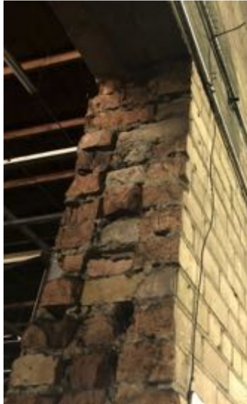
Figure 13. Unreinforced masonry wall in the EDSO portion of the building.
