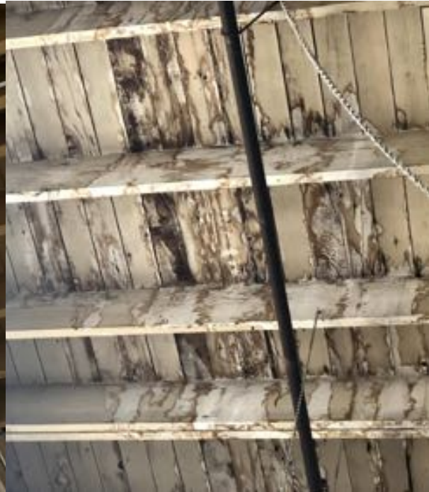
Figure 8. Potential water damage in East Building.
