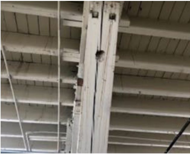
Figure 11. Split bracing in East Building.
