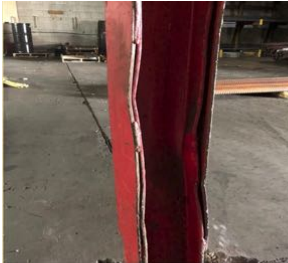
Figure 1. Damaged column in the EDSCO manufacturing facility.
