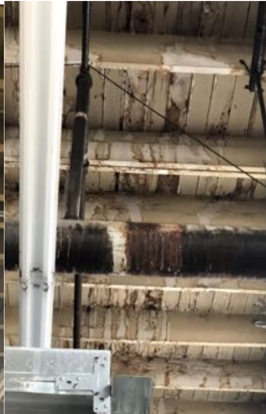
Figure 10. Potential Water Damage in East Building.
