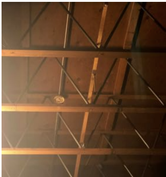
Figure 3. EDSCO open web roof structure.
