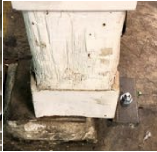
Figure 12. Displaced column in West Warehouse.
