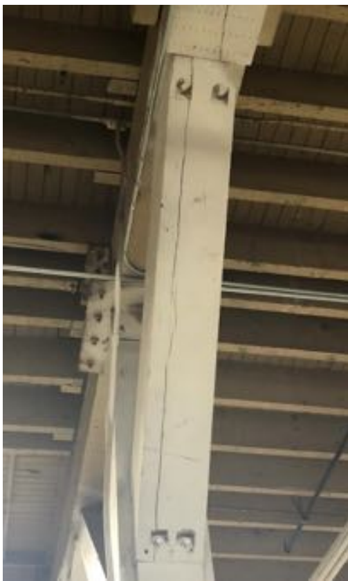
Figure 9. Split bracing in East Building.
