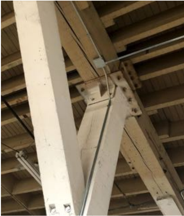
Figure 7. Split beam in East Building.
