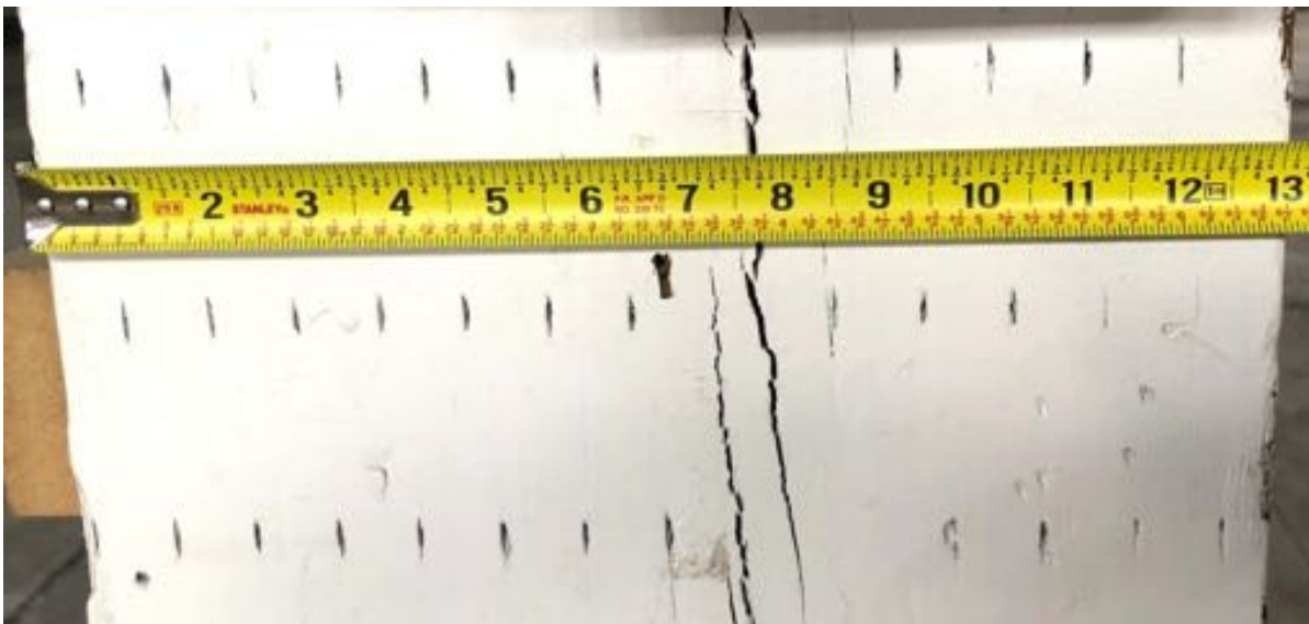
Figure 6. Split column in East Building.
