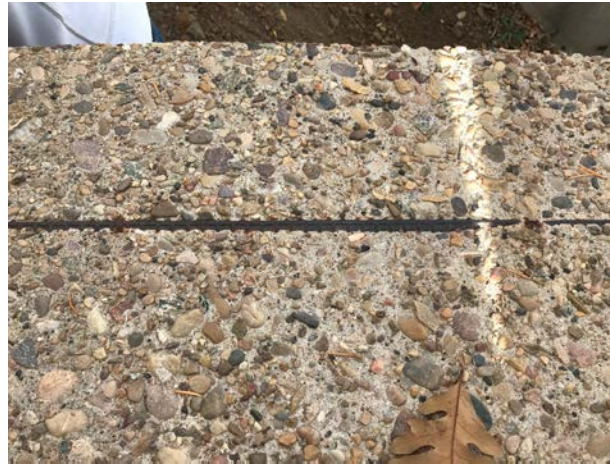
Exposed Rebar
