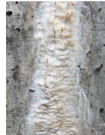
Efflorescence
