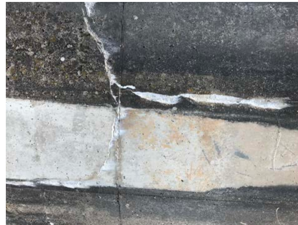
Cracking
