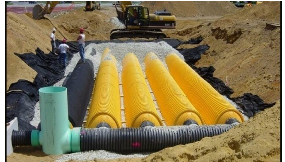
StormTech Infiltration System Installation
