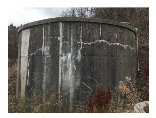
As can be seen from the pictures, the tanks are built partially into a hillside. Signs of leakage are visible on both tanks. It also appears that the tanks were built at different times, or in different manners. This is evident from small differences in lids, tank tops, color, and general condition. The north tanks appears to be newer than the south tank. This could potentially have an effect on the final decision, with the possibility of replacing only one tank.
