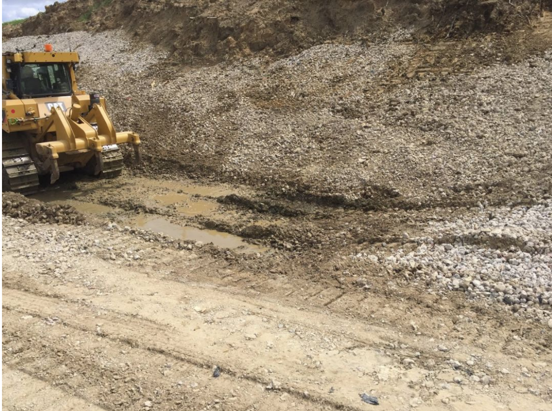
Figure 2. Bottom of Slope After Failure
