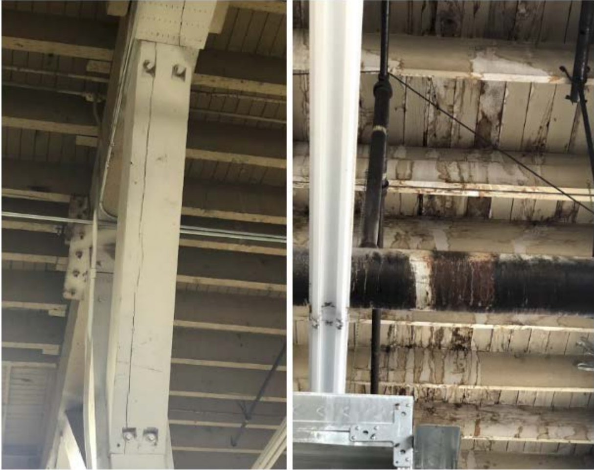
Figure 4: Split (right) and Water Damaged (left) Members
