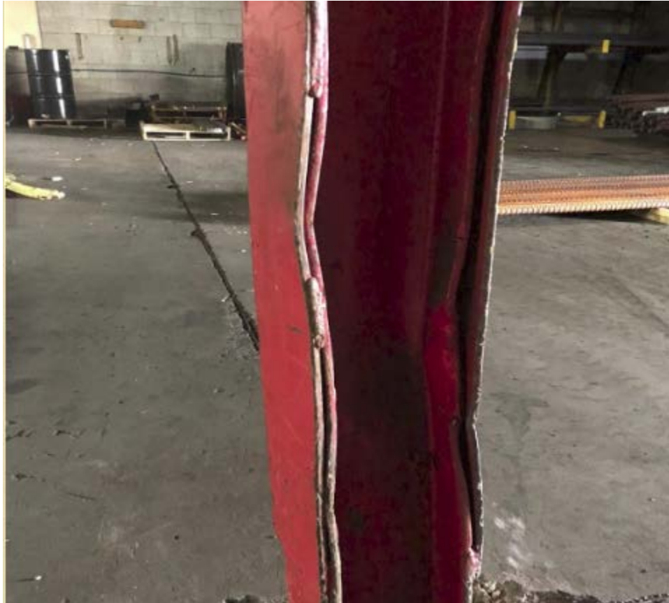
Figure 1: Damaged Columns
