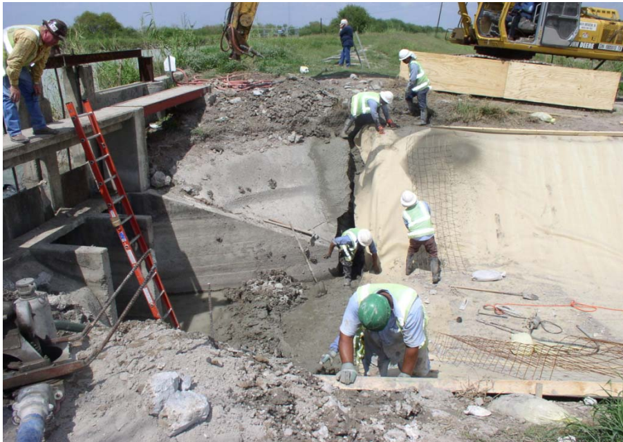
Cut-off trench excavated across the canal bottom (Concrete)
