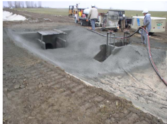
Canals with Shotcrete cover
