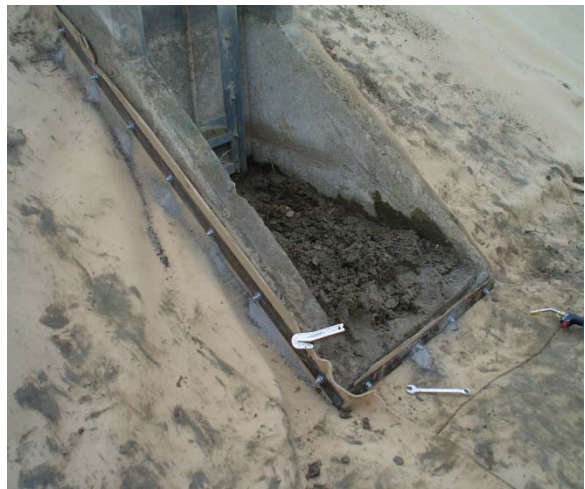
Two inch steel batten strips anchored to wall with expansion anchors on one foot spacing
