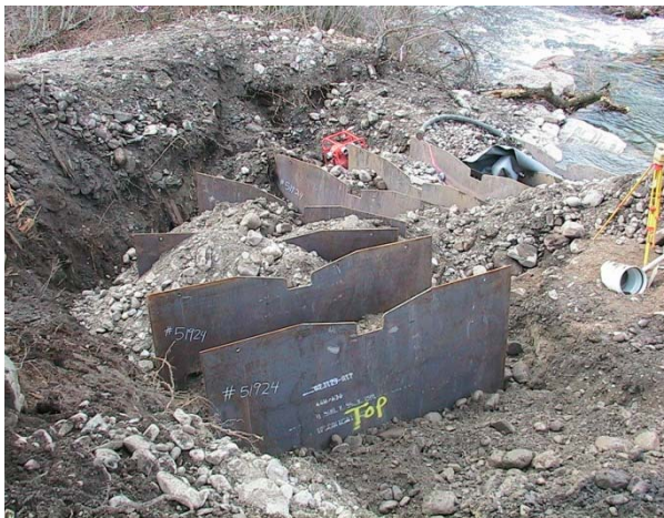
Fish Ladder Bays
