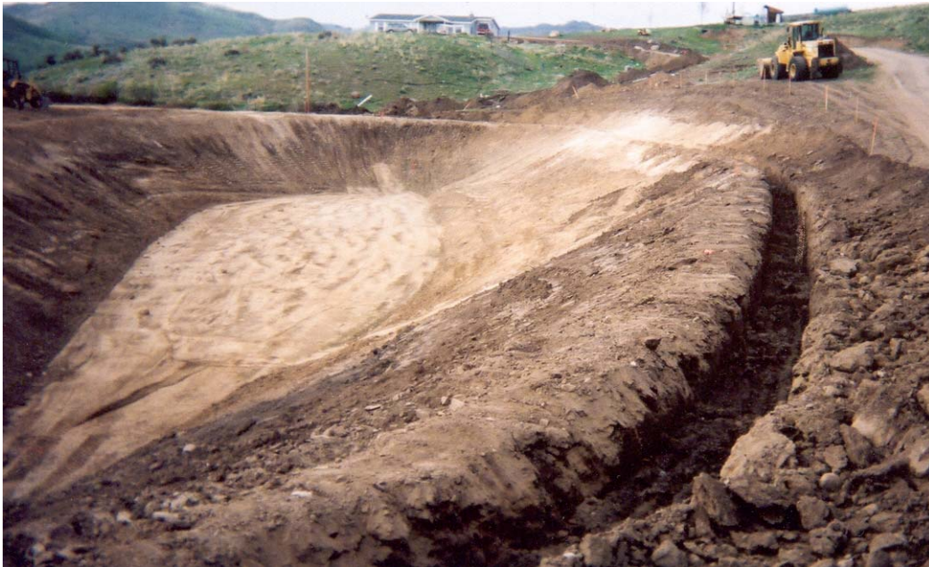
Rectangular Anchor Trench (10 – 20 ft slope)
