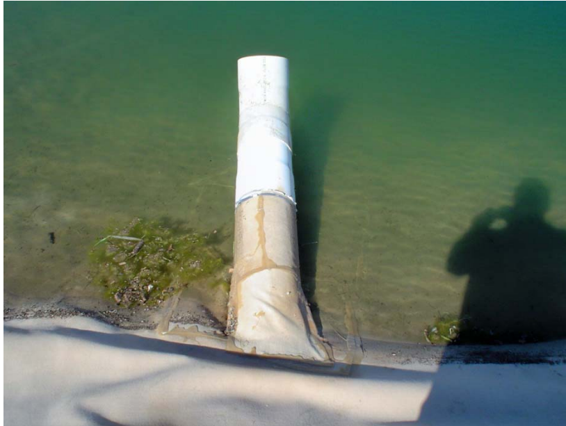
Finished boot around 12 inch PVC emergency outlet pipe
