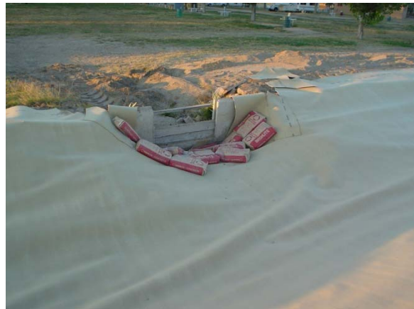
Concrete bags used to hold material down
