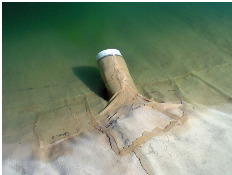
Finished boot around 10 inch PVC fill pipe
