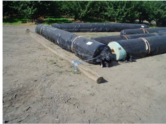
Simple lifting bars built by the irrigation districts. Minimum pipe diameter is 3 inches
