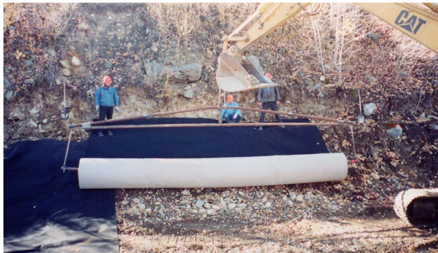
Canal 3 being unrolled across the canal
