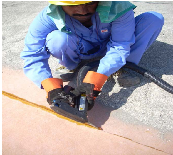
Canal 3 being seamed with a hot melt adhesive
