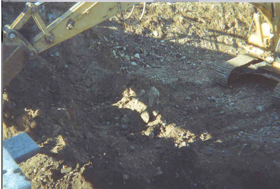
Cut-off trench excavated across the canal bottom (Earth)
