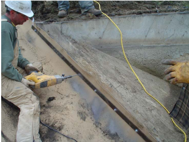
Two inch steel batten strips anchored to wall with expansion anchors on one foot spacing
