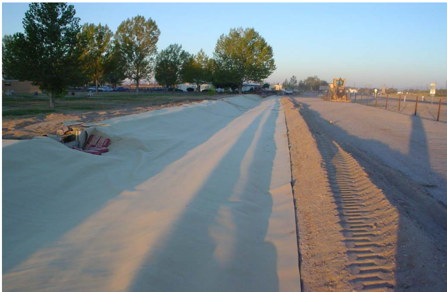
V-Anchor Trench (2 – 5 ft side slope)
