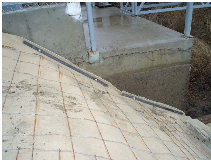
Steel batten strips anchored to wall with two expansion anchor bolts on each end
