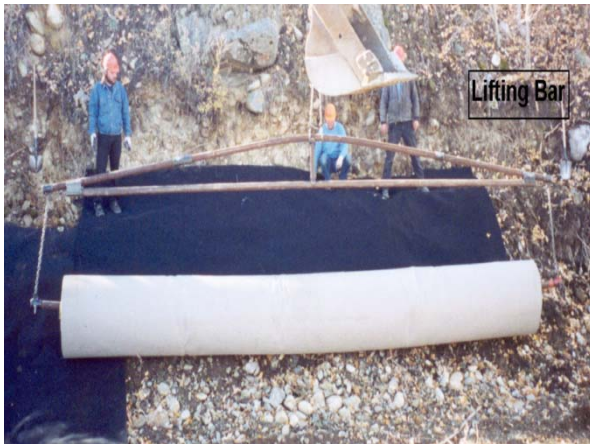
Simple lifting bars built by the irrigation districts. Minimum pipe diameter is 3 inches
