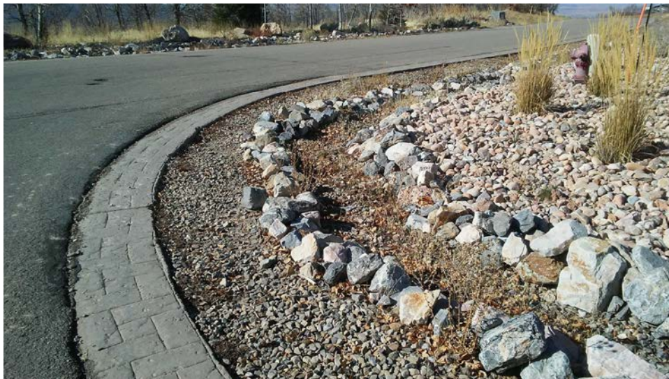
Figure 11: Existing riprap channel.
