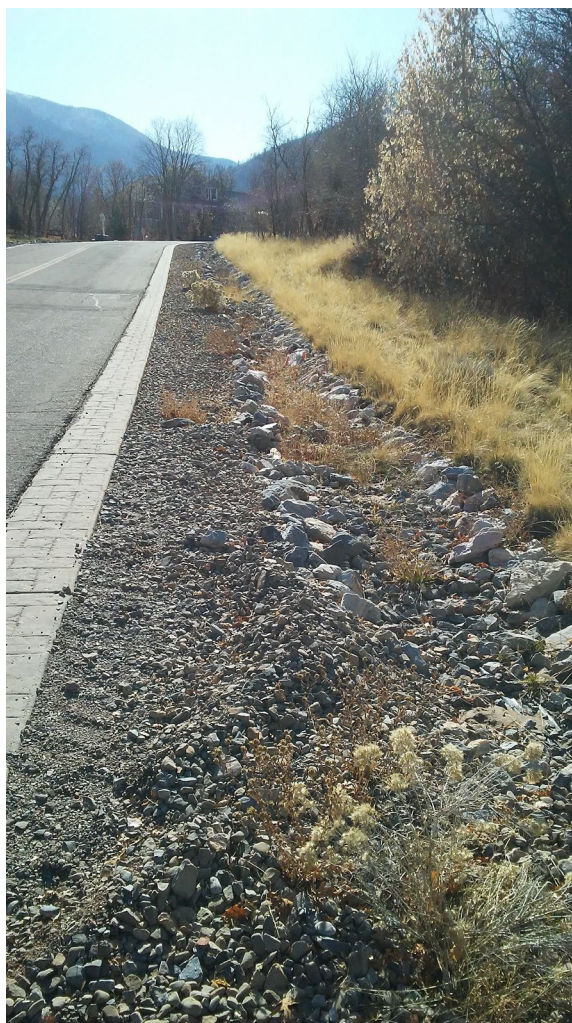
Figure 6: LID rip rap alongside a road.
