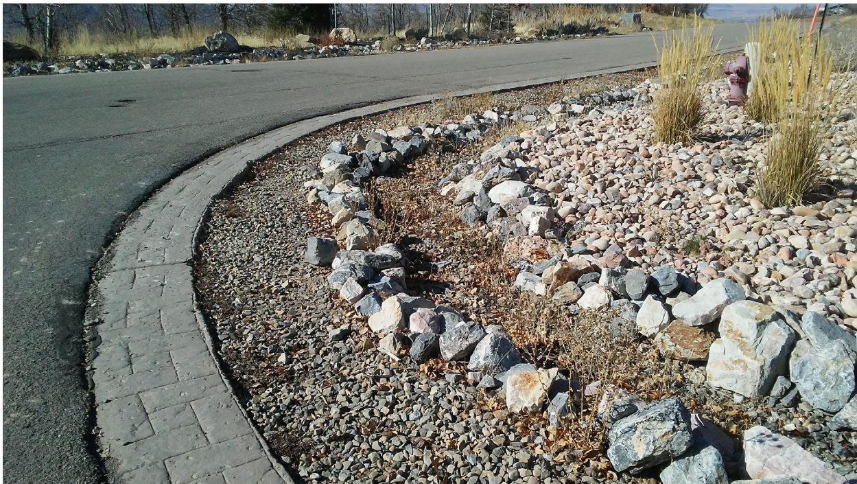
Figure 8: Rip rap alongside a culvert.
