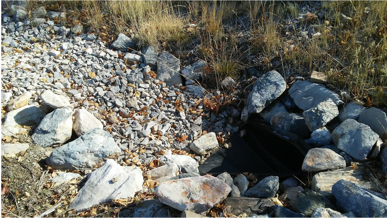
Figure 7: Rip rap going into a culvert.
