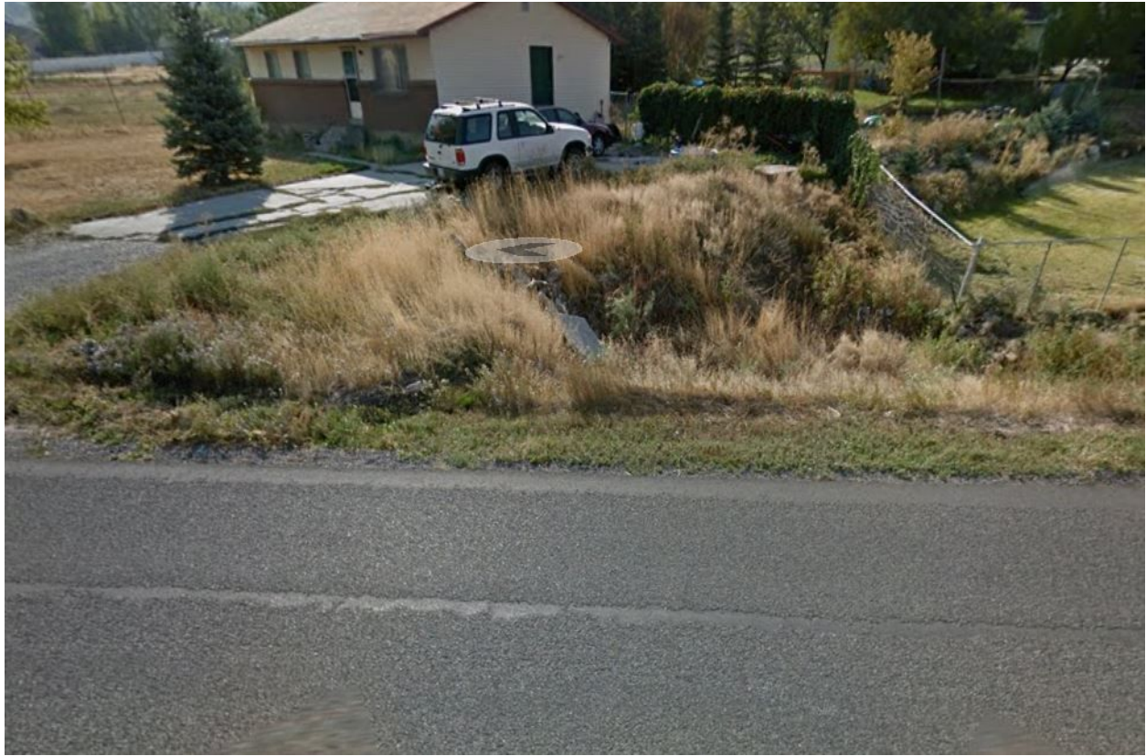
Figure 2: The depression requiring large fill or a possible boardwalk structure at 255 South Highland Drive.
