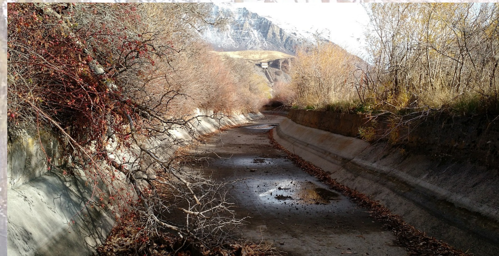
Canal segment is 3.7 miles in length
