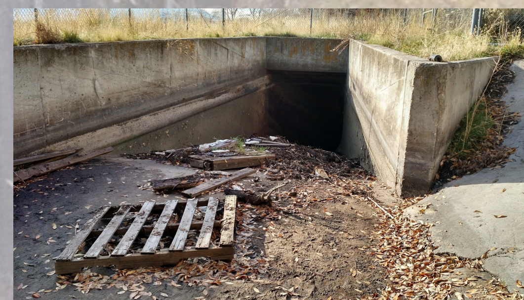
Siphon structure crossing under Orem Center Street
