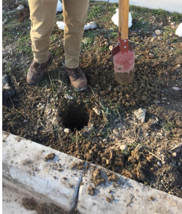
Figure 3: Hole dug for percolation tests
