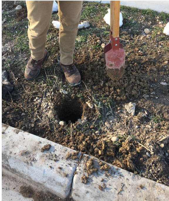
Figure 3. Hole dug for percolation tests
