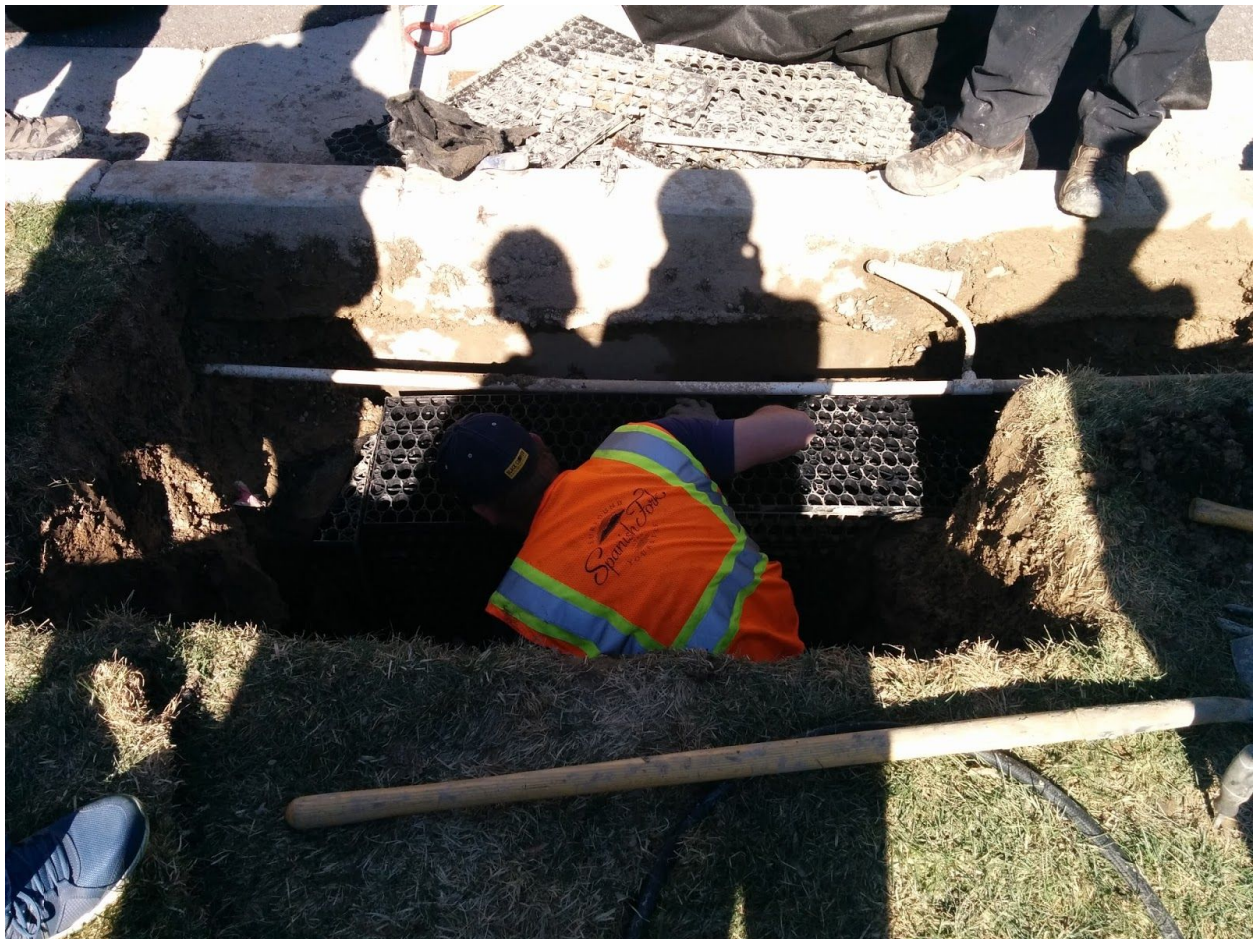
Figure 6. The excavation of the R-tank.
