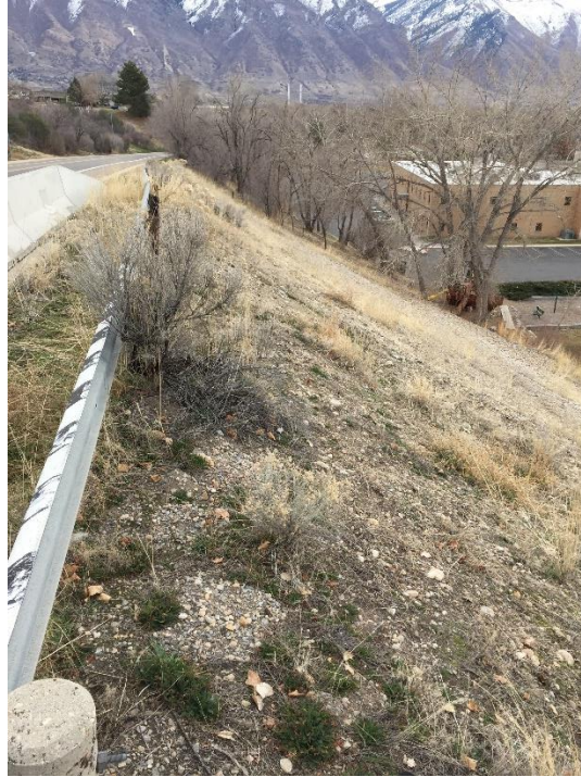
Figure 13: Hillside of the Provo City Connector
