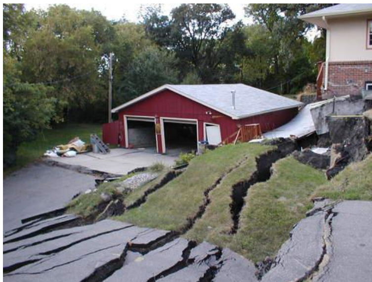
Figure 1: Landslide damage to nearby home, September 2003 (Source: www.valleynewslive.com ).
